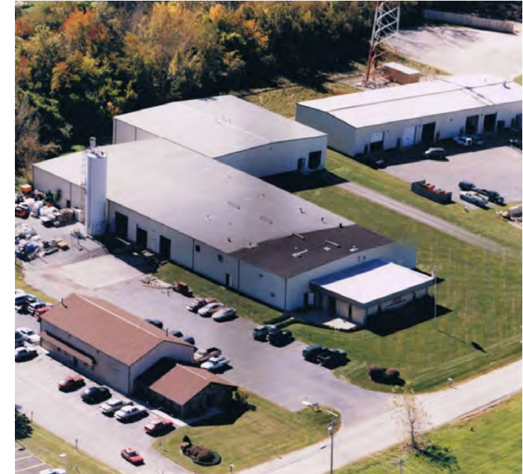
Plainfield, Indiana Facility
